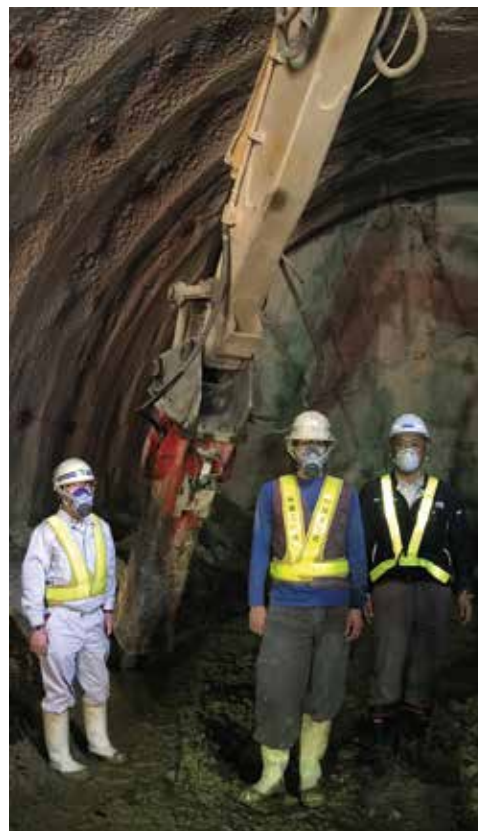
Above: Crescendo Infra is using a Rammer 5011, mounted on a 45 t class Volvo E460 excavator, to break exceptionally hard granite on a residential project in Malaysia.
