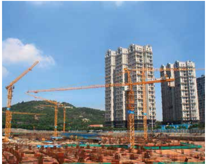
Above and bottom: Potain tower cranes work on the Haixi Jinggu Square development, which is set to be the largest financial complex in Xiamen, Fujian Province, China. The cranes are used to lift building materials up to heights of 180 m.
