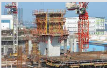
VARIO GT 24 Wall Formwork was fixed to the climbing brackets CB 240 and thus able to be lifted by crane as one unit
