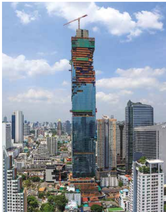
Above: The 21LC290 flat-top crane is equipped with a 110 kW hoist motor, which reaches speeds of up to 228 m/min.
