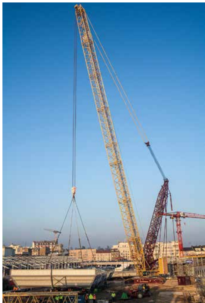
Left and right: Terex's Superlift 3800 lattice boom crawler crane helps install a footbridge over the Versailles Chantiers train station. The crane offers fast and efficient mobilisation with innovative features such as nesting boom segments and no component being wider than 3 m for transport.
