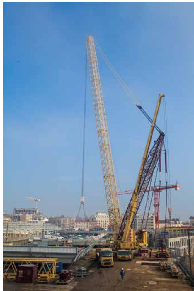
Left and right: Terex's Superlift 3800 lattice boom crawler crane helps install a footbridge over the Versailles Chantiers train station. The crane offers fast and efficient mobilisation with innovative features such as nesting boom segments and no component being wider than 3 m for transport.
