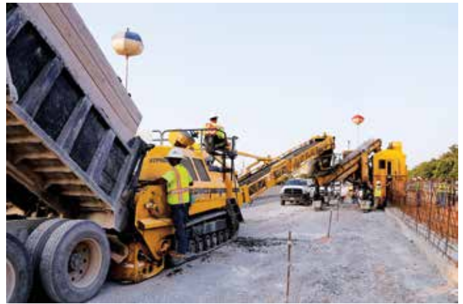
Gerdan Slipforming achieved high-production variable barrier with its Gomaco RTP-500 rubber-tracked placer and 4400 barrier paver. Production averaged 183 m per night slipforming 1,930 to 1,981 mm high wall over steel-cage reinforcing.
