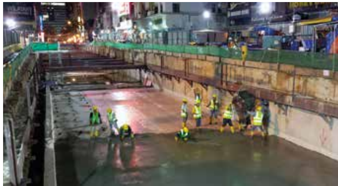
Above: Applying Purtop 1000 by spray machine.
