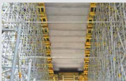
PERI UP Rosett Tableforms under the beams enabled the jobsite to avoid the usage of intermediate supports under the slab
