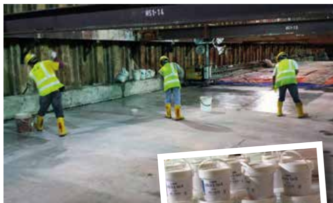
Above: Applying Biblock, a water-based epoxy curing membrane (inset), by roller.
