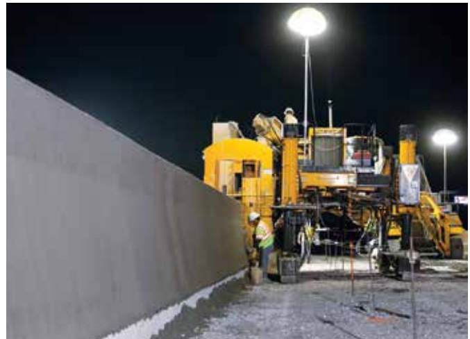
The mould required 1.5 cu m of concrete to fill, had 914 mm of variable height adjustment on each side and could reach a wall height as tall as 2 m.
