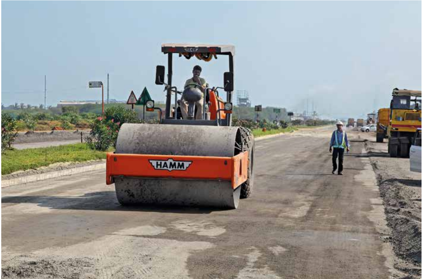
Subsequent compaction with the Hamm 311 compactor.
