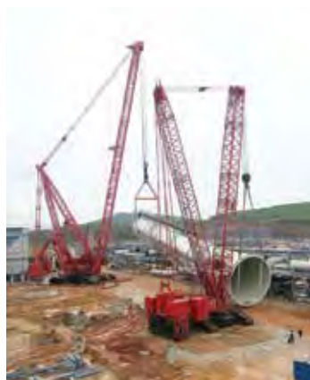
ABOVE: Manitowoc crawler cranes perform heavy lifting at a petrochemical refinery in Vietnam.
