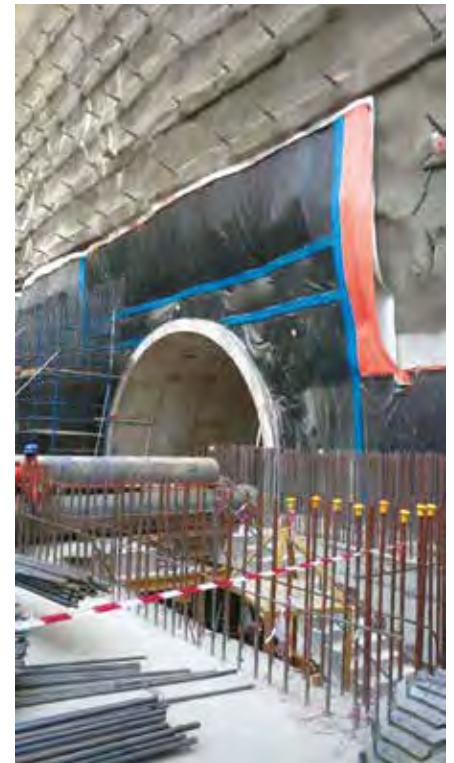
LEFT: The tension anchors posed an immense challenge to the designers when accommodating the waterproofing system. To overcome this, Mapei found an innovative solution to treat the anchors using Mapeplan TU S 20, Mapegel UTT and Planigrout 300 ME PCT.
