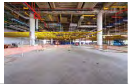
ABOVE IMAGES: A total of 2,829 precast elements covered 70 percent of the second-storey main terminal building, including precast columns, precast main and secondary beams, and precast planks.
