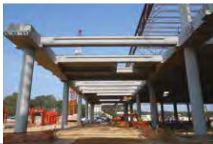
ABOVE IMAGES: A total of 2,829 precast elements covered 70 percent of the second-storey main terminal building, including precast columns, precast main and secondary beams, and precast planks.
