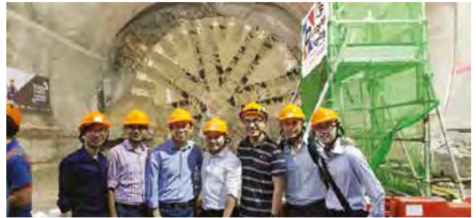
The project team celebrates the TBM breakthrough at the Lung Shan Tunnel northbound section of the Liantang - Heung Yuen Wai boundary crossing facility.
