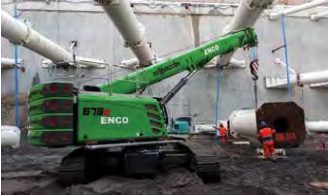
Sennebogen 673 E telescopic crane works on the Grand Paris Express project.
