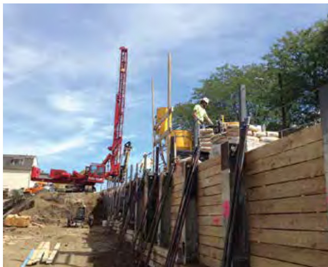
TOP: ChemGrout's CG-680 high-pressure, high-capacity, skid-mounted colloidal grout machine is designed for mixing and pumping slurries of cement, fly ash, bentonite and lime flour.
