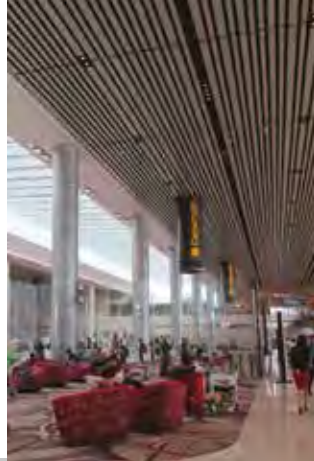
The 18.5 m large-span cantilever roof at the departure kerbside (left) and the 60 m large-span column-free roof at the departure hall were among the challenges faced by RSP.
