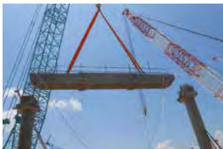
ABOVE IMAGES: A total of 2,829 precast elements covered 70 percent of the second-storey main terminal building, including precast columns, precast main and secondary beams, and precast planks.
