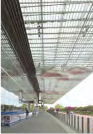
The 18.5 m large-span cantilever roof at the departure kerbside (left) and the 60 m large-span column-free roof at the departure hall were among the challenges faced by RSP.
