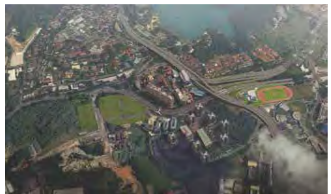
Samsung C&T has won another contract for the North-South Corridor project in Singapore, comprising a 1.7-km-long underground road and facility building in the Toa Payoh area.
