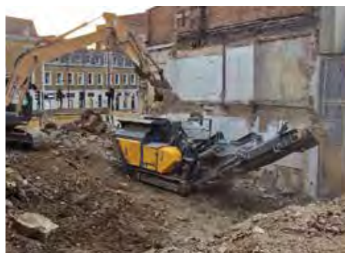
ABOVE AND LEFT: The RM 70GO! 2.0 crushes 125 t/hr quietly with low emissions near the Camden Market in London. The machine can easily drive through narrow gateways and restricted areas.
