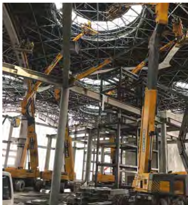
ABOVE, FAR LEFT AND LEFT: Acarlar Makine has supplied more than 300 Haulotte aerial platforms to the Istanbul New Airport project. The machines range from an electric scissor lift with an 8-m working height to the biggest diesel boom lift with a 43-m working height.
