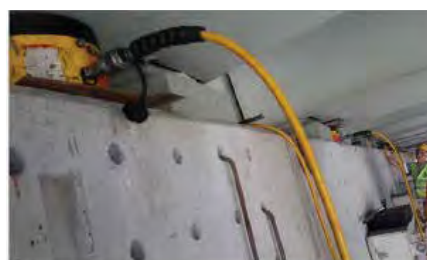
ALL IMAGES: Enerpac offers its range of high tonnage cylinders (HTC) to meet the rising demand for heavier lifts in harsher environments. The Summit Edition cylinders provide excellent durability, longer service life, and greater side load resistance for increased heavy lift capability.
