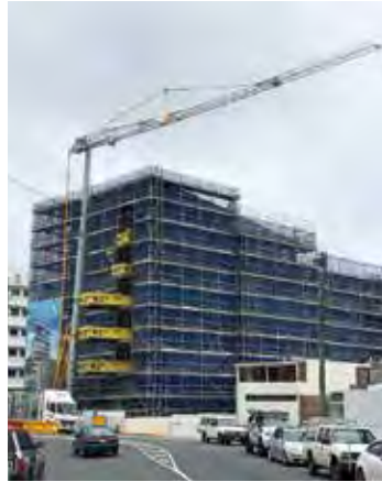
ABOVE: Many countries in Asia Pacific are now adopting the precast construction method. Here, Potain tower cranes with a high capacity are being used to lift heavy precast components on a residential project in Singapore.
