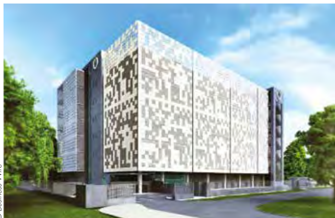
Global Switch's new data centre in Singapore will adopt the prefabricated mechanical and electrical and plumbing (MEP) modular technique.
