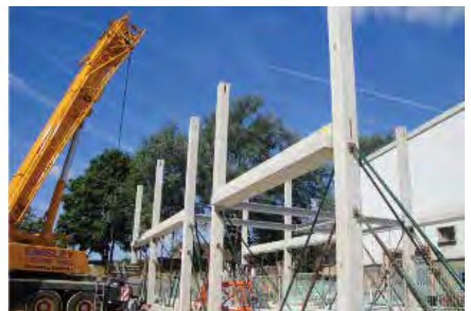
ABOVE AND RIGHT: The BSF range of Invisible Connections is designed for transferring heavy loads from beams into columns, walls or other beams. These three-part telescopic connectors have individual capacities ranging from 225 to 700 kN.
