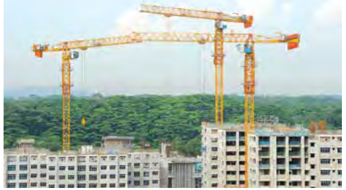
ABOVE: Many countries in Asia Pacific are now adopting the precast construction method. Here, Potain tower cranes with a high capacity are being used to lift heavy precast components on a residential project in Singapore.
