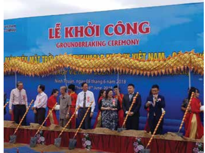
The groundbreaking ceremony for the construction of a new US$150 million solar power plant in Ninh Thuan, Vietnam, was held in June 2018. This 168-MW facility is expected to reach commercial operation by June 2019.
