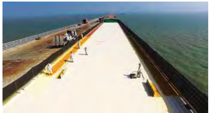
The Eliminator bridge deck waterproofing system from GCP Applied Technologies being used on the project. This cold-spray-applied system is fast, effective and able to seal complex, critical details and penetrations with ease.
