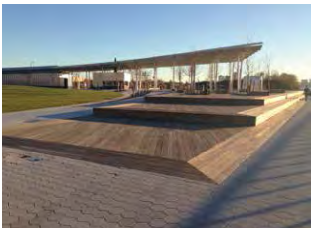
Kebony decking at the Hunter's Point South Waterfront Park in New York.
