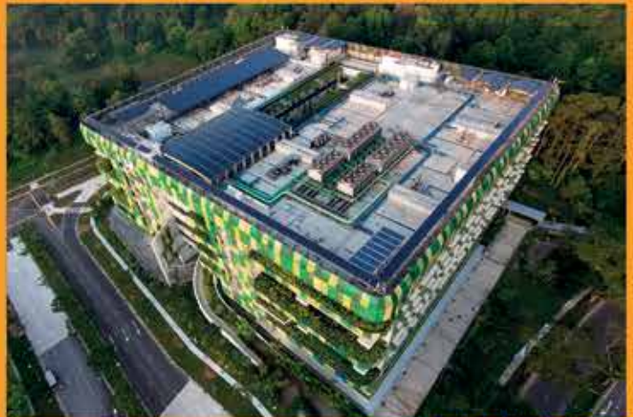
Commercial Rooftop - 2.31kWp, Singapore
