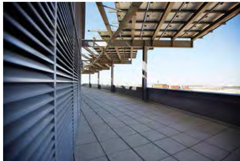
A 1,000 square metres solar photovoltaic rooftop system will produce 305,000 kWh of electricity annually. Photo: © International Renewable Energy Agency (IRENA)
