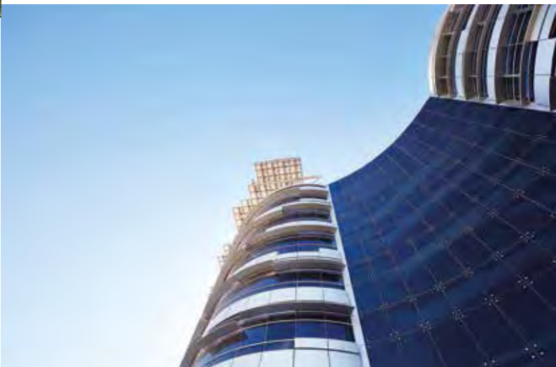
Thanks to an efficient envelope, the building is twice as airtight as Estidama requires, reducing overall energy use. Photo: © International Renewable Energy Agency (IRENA)
