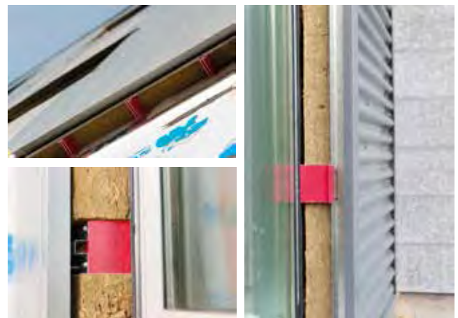
The Cascadia Clip® cladding support system. Photos: © Paul Grdina
