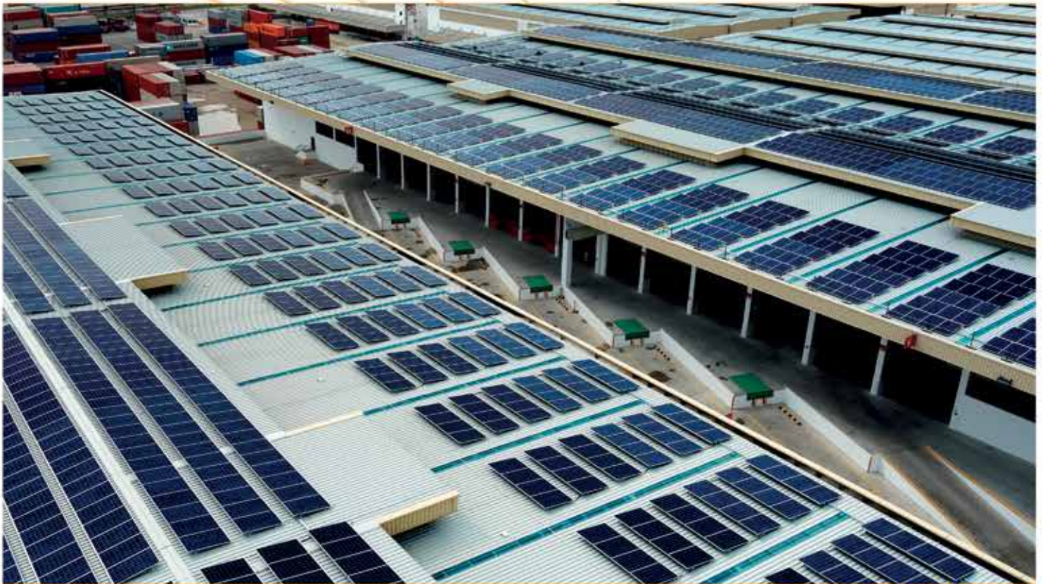
Industrial Rooftop - 1.188kWp, Singapore
