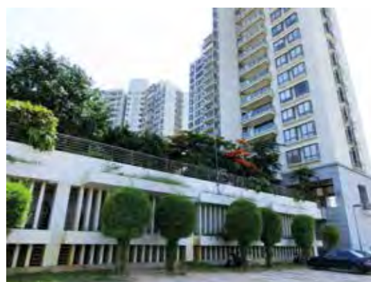
Fig 9: The roof garden is built at level 2, on top of the car parking deck.
